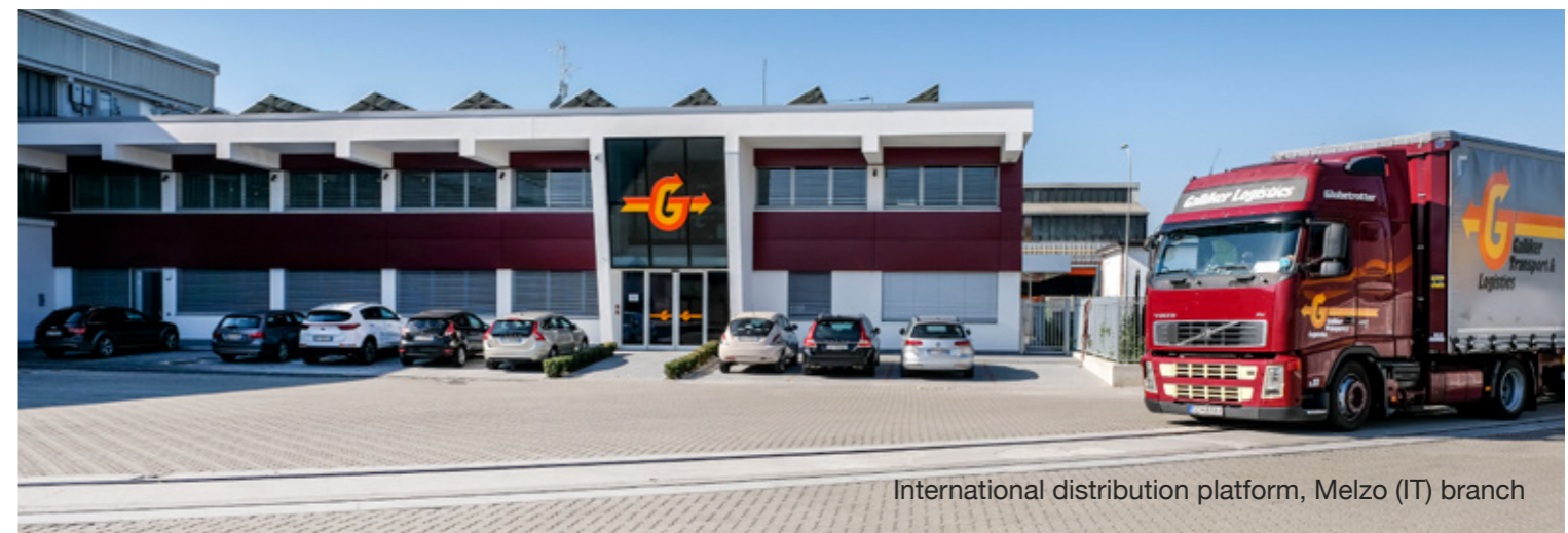
Logistics Centre 4, Dagmersellen
